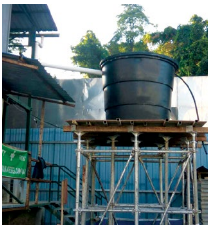
Simple harvesting systems collect rainwater for general cleaning - one of the on-site activities that consumes the most water.
