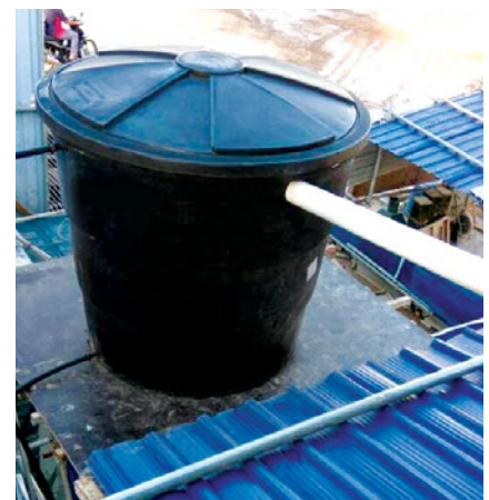
Simple harvesting systems collect rainwater for general cleaning - one of the on-site activities that consumes the most water.
