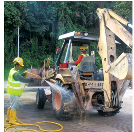
Washing bays provide quick and effective cleaning so heavy vehicles do not track mud and silt.
