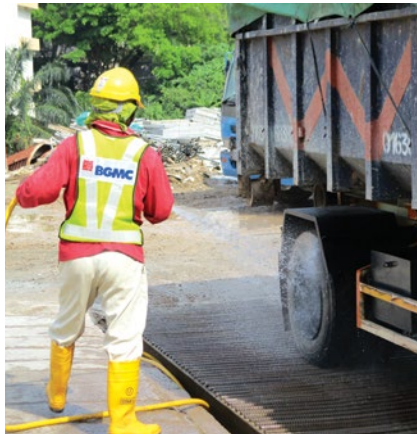
Washing bays provide quick and effective cleaning so heavy vehicles do not track mud and silt.
